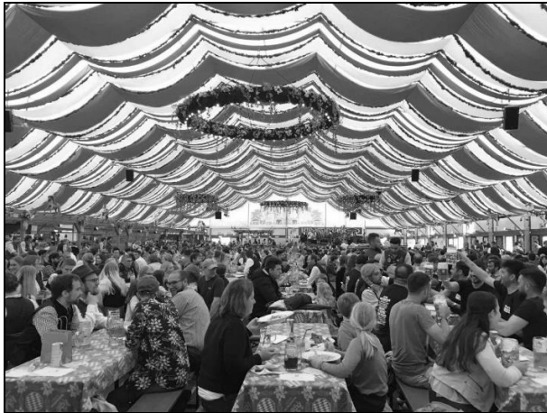
Fig. 2. Awning structure of Oktoberfest in Munich
